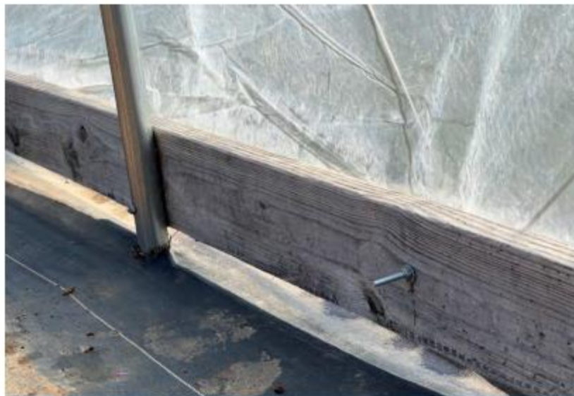
Photo 5.4 Many tunnels use wood in addition to metal for their structure. Wood components can wear down and get damaged. The easiest time to fix them is when you have the plastic off the tunnel for replacement. Source: Kathryn Pettigrew
